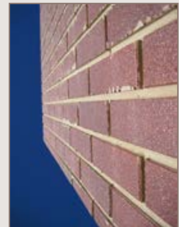
Partially stripped, but not yet cleaned panel using Versaliner MP
