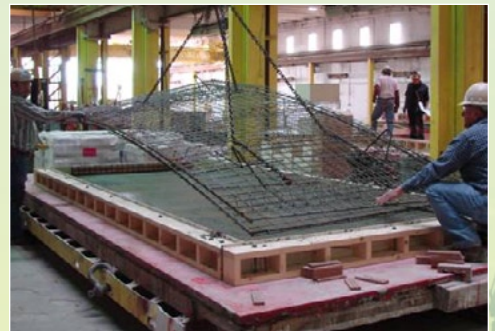
Cage being placed.
